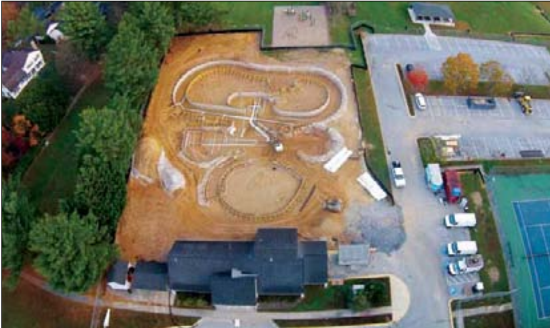
Work is progressing on the Apple Ridge Pool Renovation. The site has been regraded and pool walls have been shaped with forms. Underground piping and other work is being set before the pool is ready for concrete. Concrete work is expected to be finished before the end of the year.
