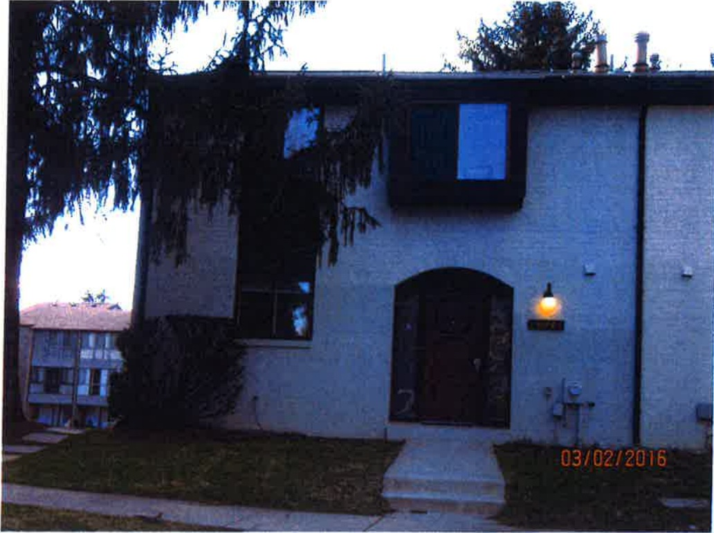
18944 Montgomery Village Avenue
