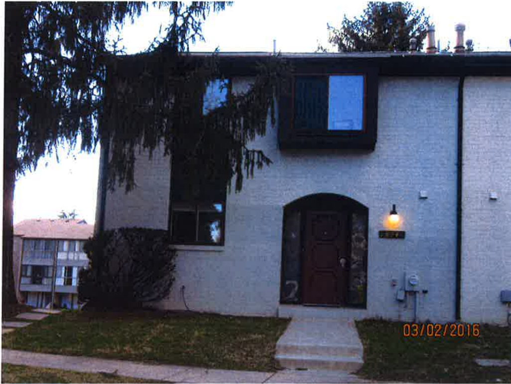
18944 Montgomery Village Avenue
